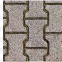
INTERNAL ROADS INTERLOCKING BLOCKS/ TREMIX CONCRETE ROAD
