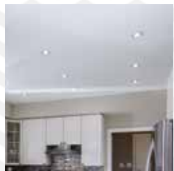
WALL / CEILING OIL BOUND DISTEMPER
