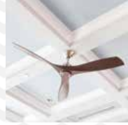
CEILING OIL BOUND DISTEMPER
